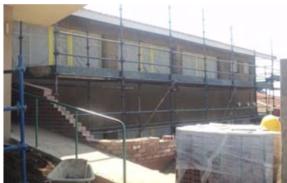
Phase 1: Soon to be finished temporary Admin. Offices
