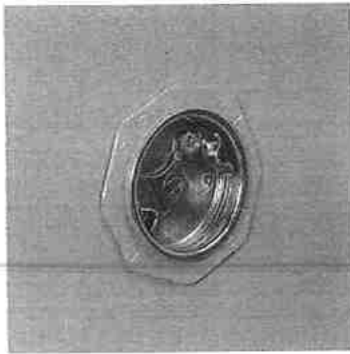
fireproofing ventilation hole
