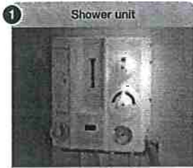
1 Shower unit The shower unit has a thermo-static mixer and temperature display.
