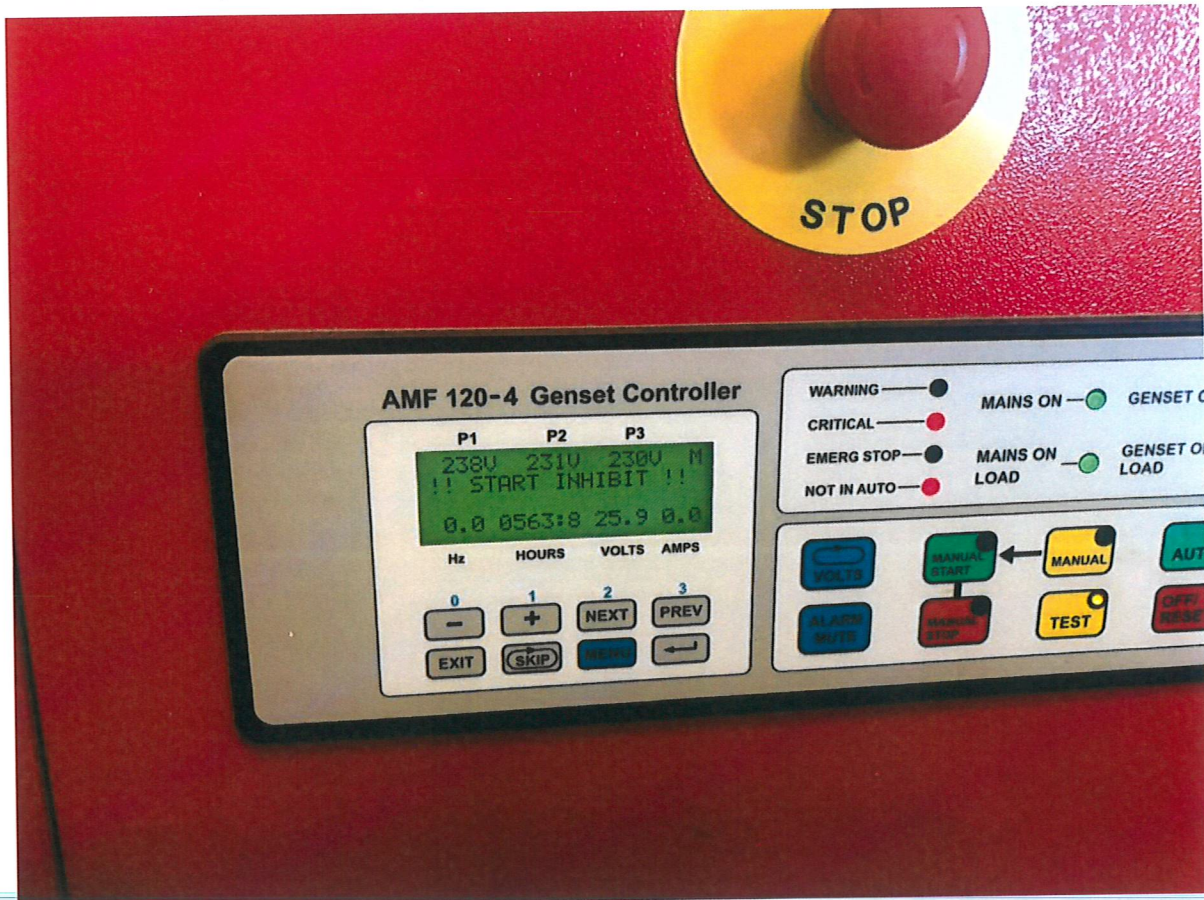
Critical fault alarm when the genset is starting up which needs urgent attention
