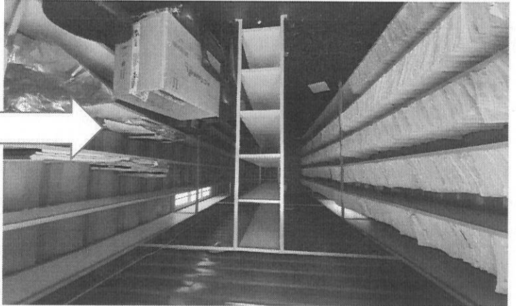
Steel shelving fixed to walls and center rack braced for
