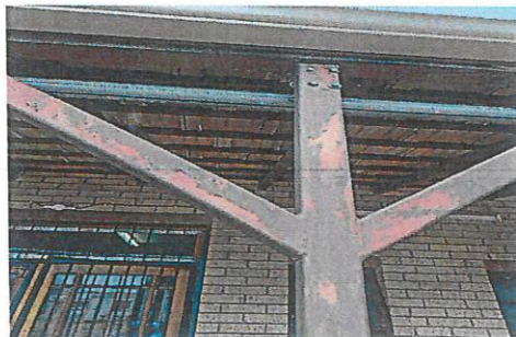
Y shaped roof support
