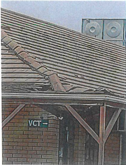
Collapsing roof
