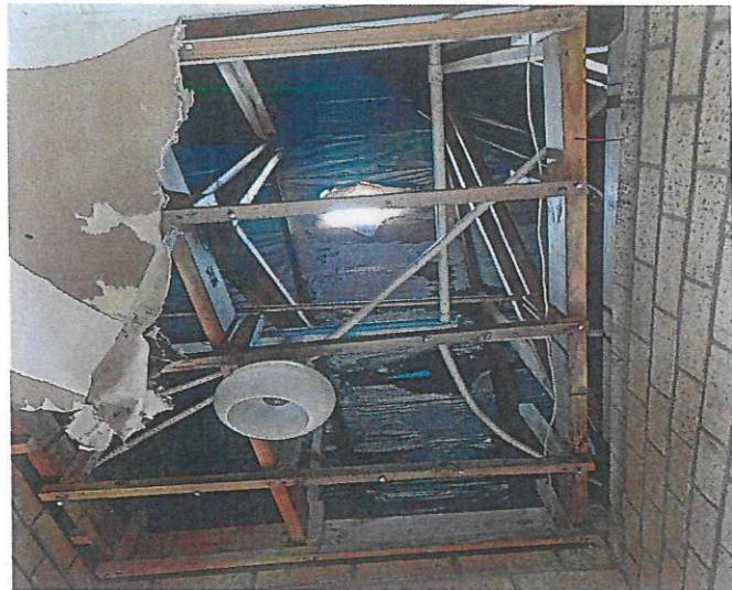
Damaged ceiling
