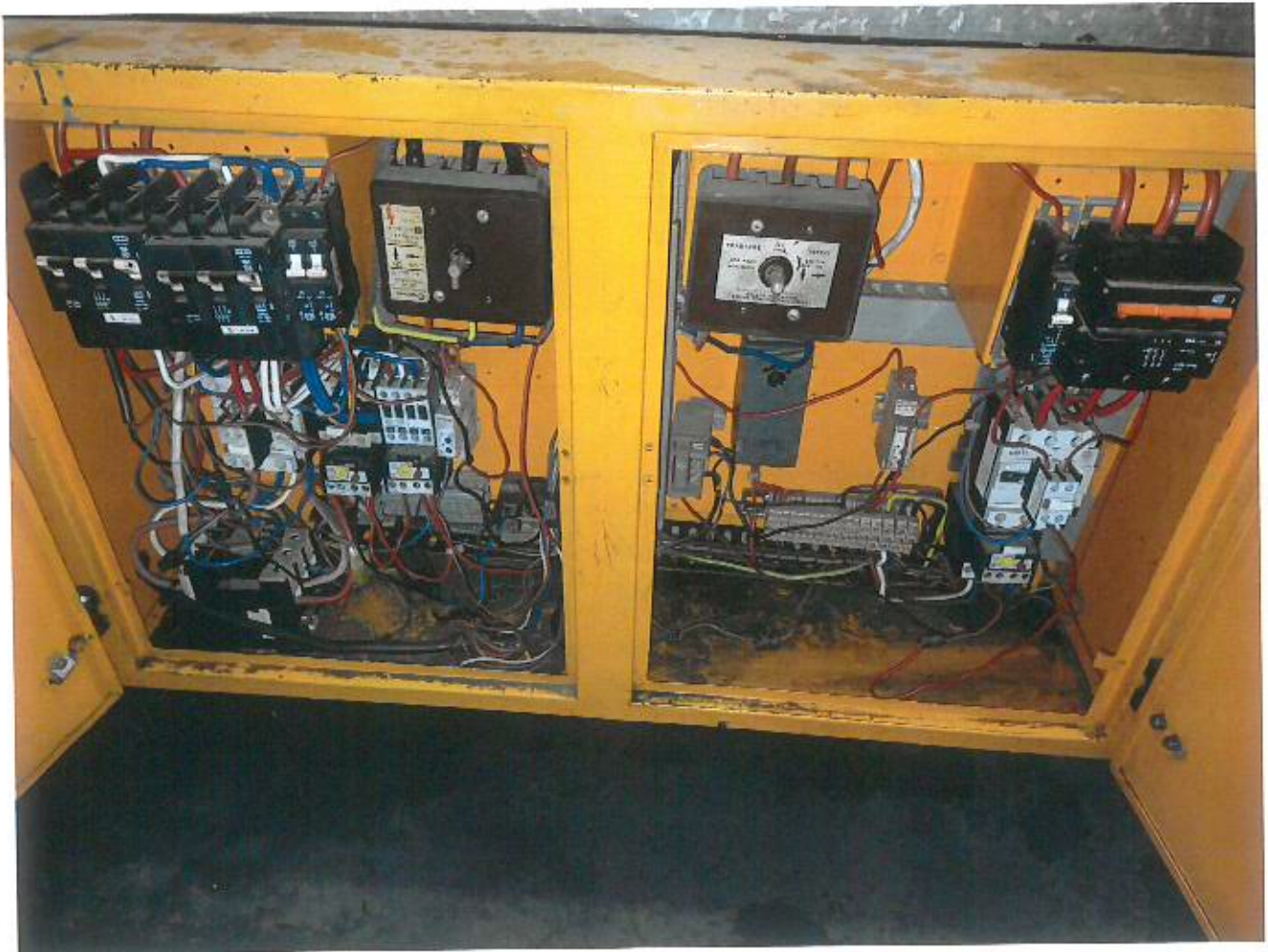
SPASSETTI WIRING
