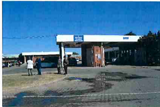
Fig 30 & 31: Existing access to wash area. No proper drainage for water. Water surface drain
