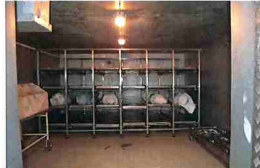
Fig 24 & 25: Existing interior of mortuary and typical fridge interior. No compartmentalized shelving provided.
