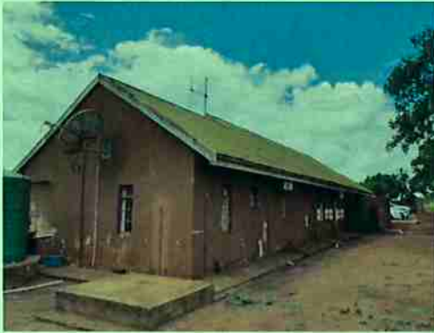
Photo 5 View of exterior of Clinic Block
