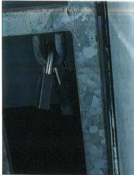
Pictures 7 & 8: Shows burglar bars that are permanently locked and obstruct the evacuation and/or escape routes. This has been flagged by the EThekwinl Metro's Fire Department as dangerous as it will severely obstruct the safe and quick evacuation of staff, patients and visitors.
