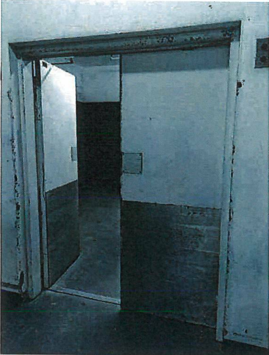
Pictures 5 & 6: Shows bump plates on fire doors that are in a very poor condition. The proposal is to replace all these with a thicker gauge aluminum material
