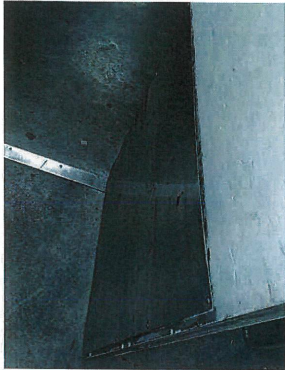
Pictures 5 & 6: Shows bump plates on fire doors that are in a very poor condition. The proposal is to replace all these with a thicker gauge aluminum material
