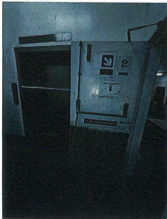
Pictures 1 & 2: Shows dilapidated fire door where repairs can be done but the 2Hr fire resistivity cannot be guaranteed. Slam bars that are completely damaged and unrepairable
