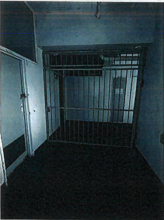
Pictures 7 & 8: Shows burglar bars that are permanently locked and obstruct the evacuation and/or escape routes. This has been flagged by the EThekwinl Metro's Fire Department as dangerous as it will severely obstruct the safe and quick evacuation of staff, patients and visitors.
