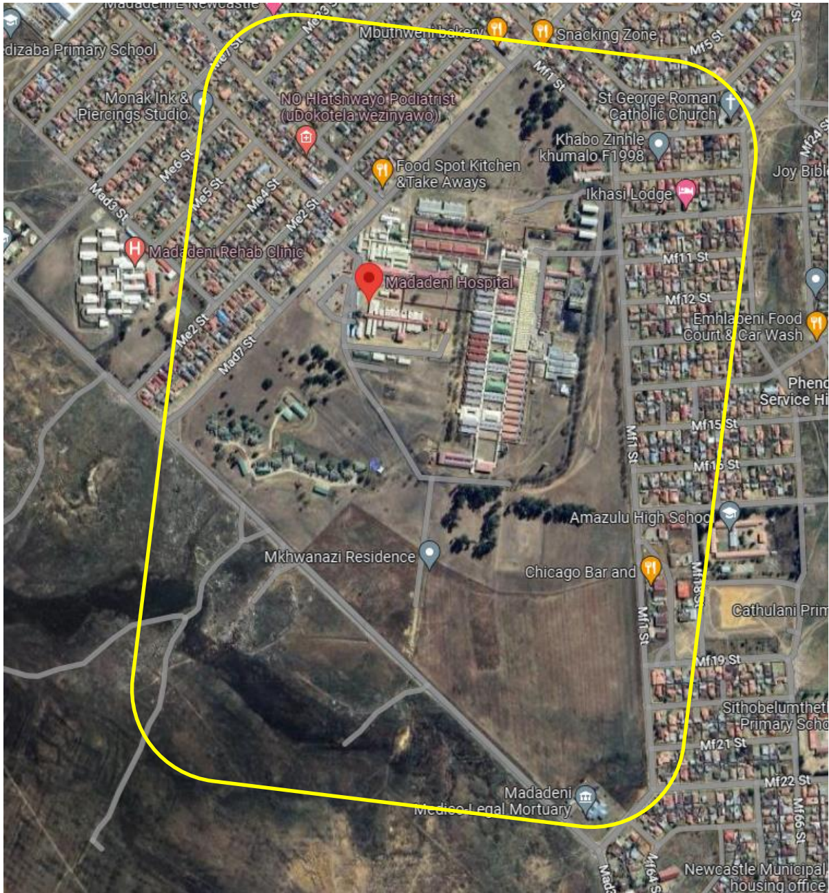
Aerial View 1: Madadeni hospital
