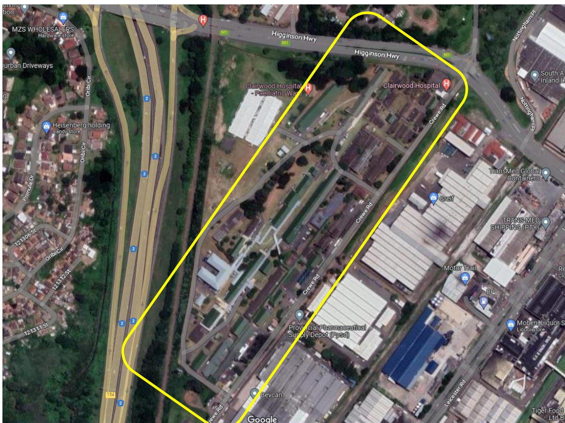
Aerial View 1: Clairwood hospital
