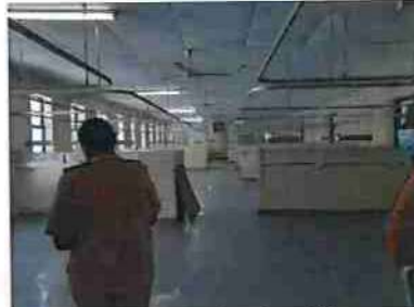
Image 2 Ward Interior Condition
