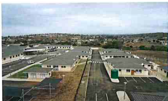
Photo 5: Othobothini CHC entrance
