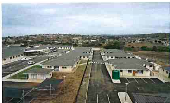
Photo 5: Othobothini CHC entrance
