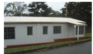
One of two new accommodation block
