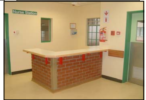
This is a new ward nursing station. It has been upgraded to meet new standard
