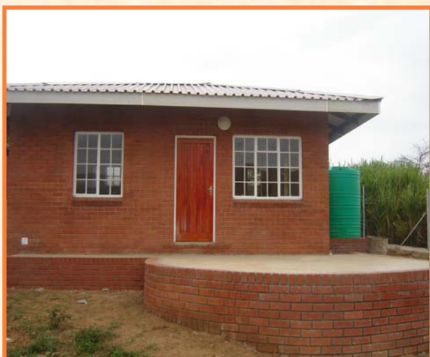
Newly constructed nurses home
