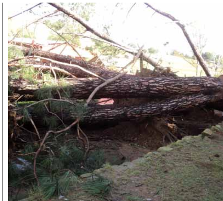
The main entrance to the hospital after the storm
